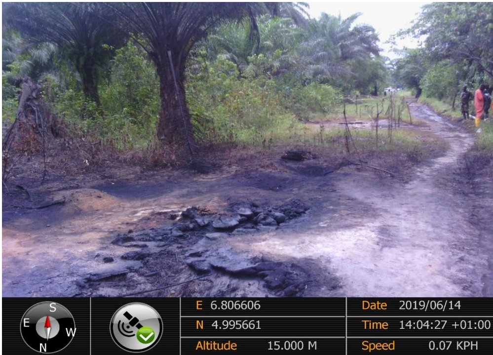
Overview: Part of spill impact on 4" Obele – Ibaa Pipeline Right of Way at Ibaa Picture was taken during Joint Investigation of 14 th June 2019.
