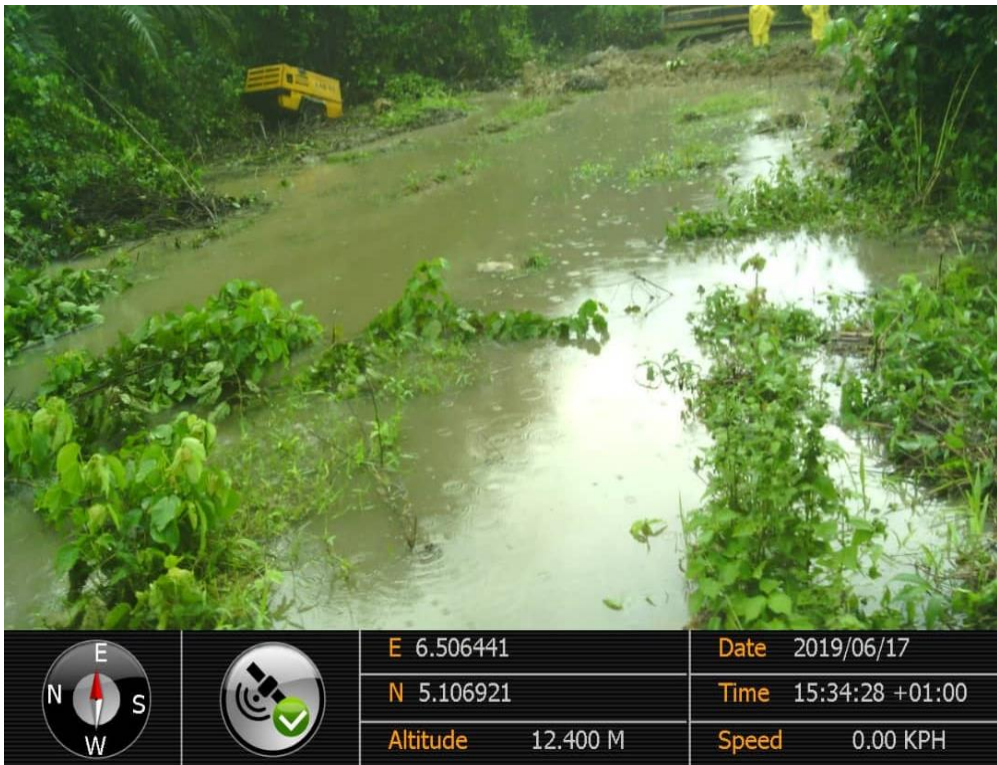
Overview: Part of spill impact on 14" Okordia – Rumuekpe Pipeline Right of Way at Oshie. Picture was taken during Joint Investigation of 17 th June 2019.
