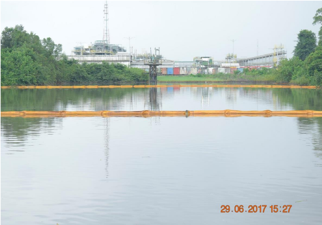
Overview: Booms enclosing Tunu Well 7T Wellhead Slot at Agbidiama. Picture was taken during Joint Investigation of 29 th June 2017.
