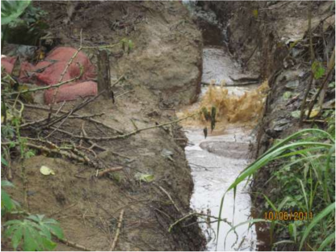
Overview: Part of the spill impact on Obigbo Well 28LS flowline at Imea. Picture taken during Joint Investigation of 10 th June, 2011
