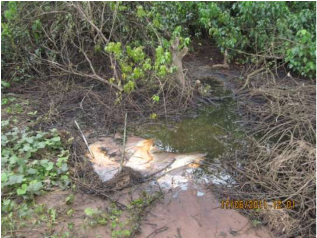
Overview: Part of spill impact on 12" ImoRiver2 pipeline at Odagwa. Picture taken during Joint Investigation of 17 th June, 2011
