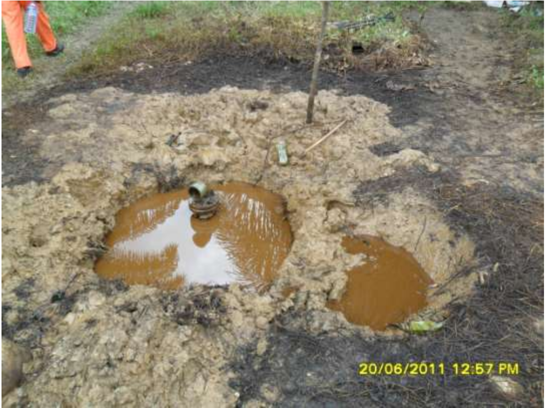
Overview: Part of the spill impact on Okordia-Rumuekpe pipeline and Akalamini riser at Akalamini. Picture taken during Joint Investigation of 20 th June, 2011
