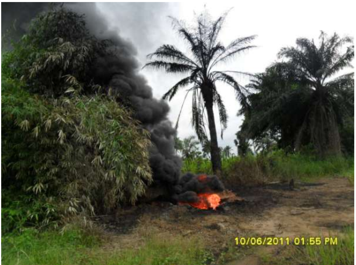
Overview: Another view of fire on 24" Bomu-Bonny Pipeline at Bodo (Ogoni).
