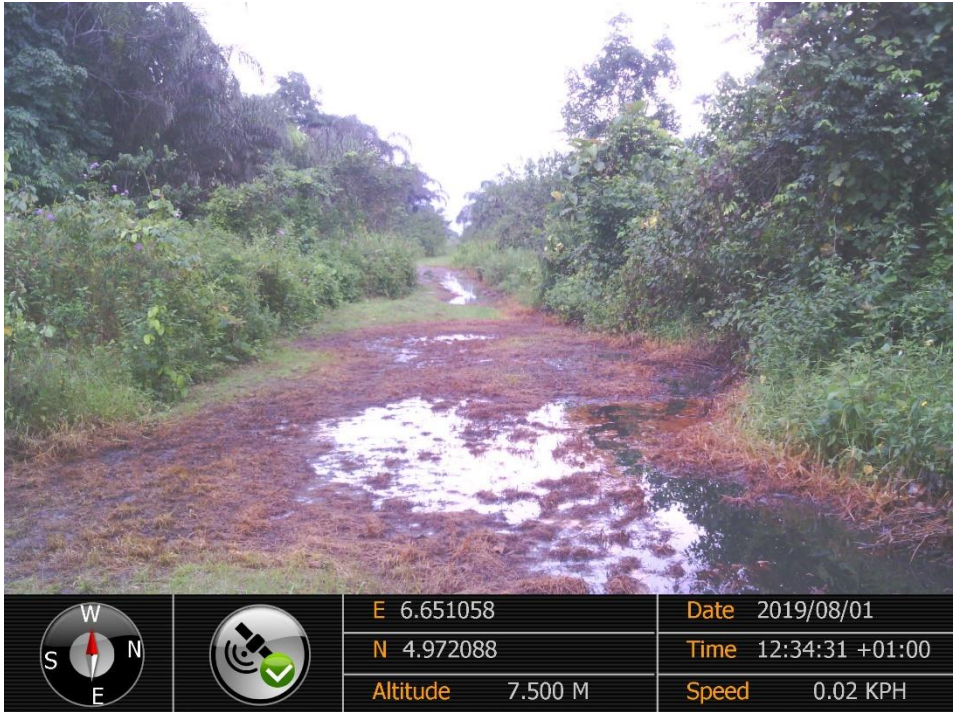
Overview: Part of spill impact on 20'' Kolocreek - Rumuekpe Pipeline Right of Way at Okoma. Picture was taken during Joint Investigation of 1 st August 2019.
