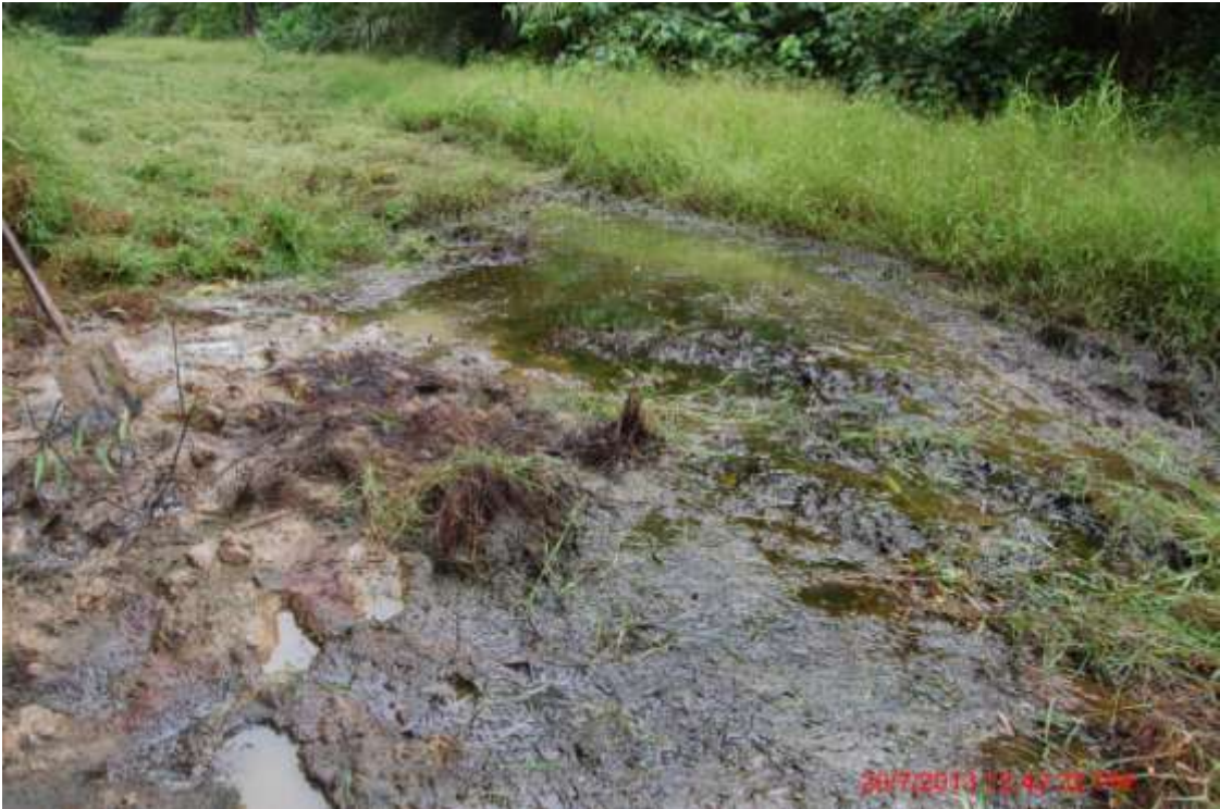
Overview (Point B) : Part of spill impact on 12" Adibawa-Okordia pipeline right of way at Ikarama. Picture was taken during Joint Investigation of 20 th July 2013.
