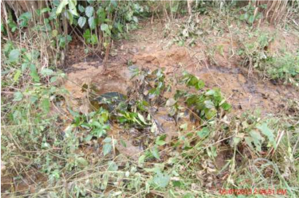
Overview: Part of spill impact 6" Obigbo North – Ogale pipeline right of way at Ogale. Picture was taken during Joint Investigation of 5 th July 2013.
