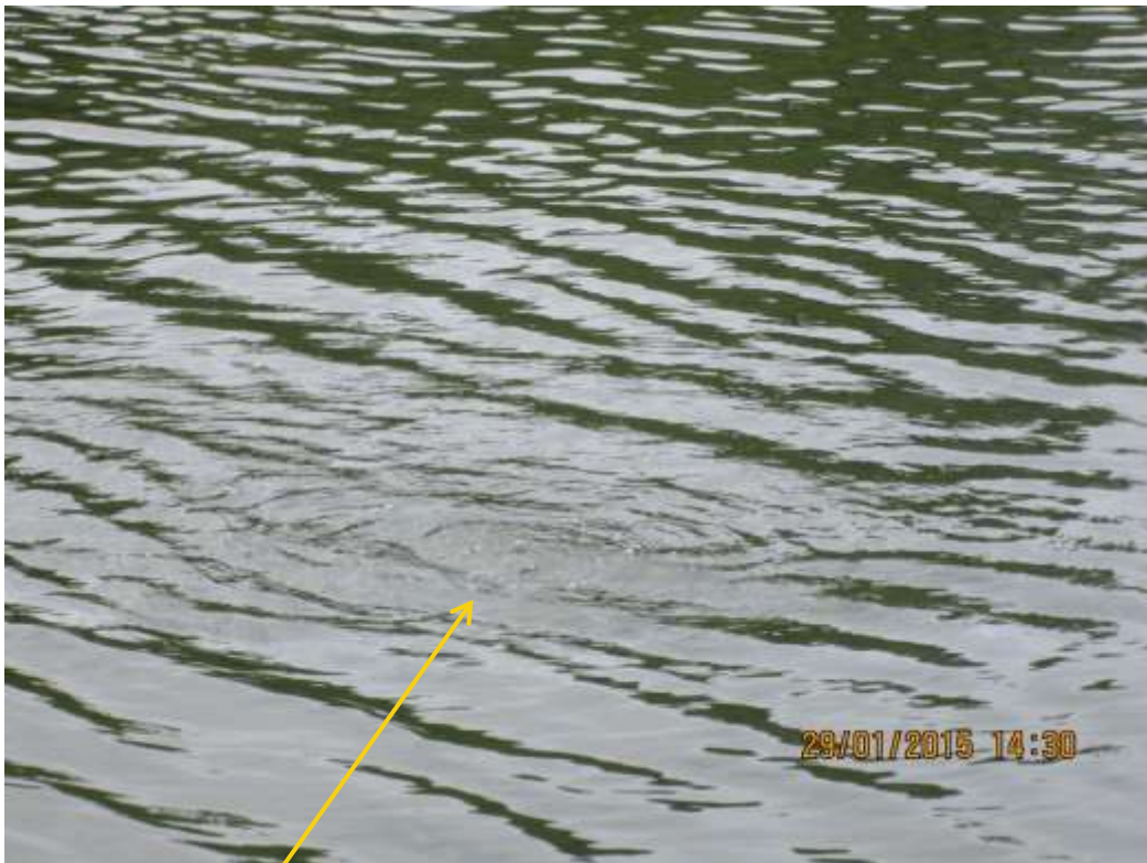
Close-up: Bubbles observed at spill point on Nembe1 Well11L 4" Flowline at Nembe Creek. Picture was taken during Joint Investigation of 29 th January 2015.
