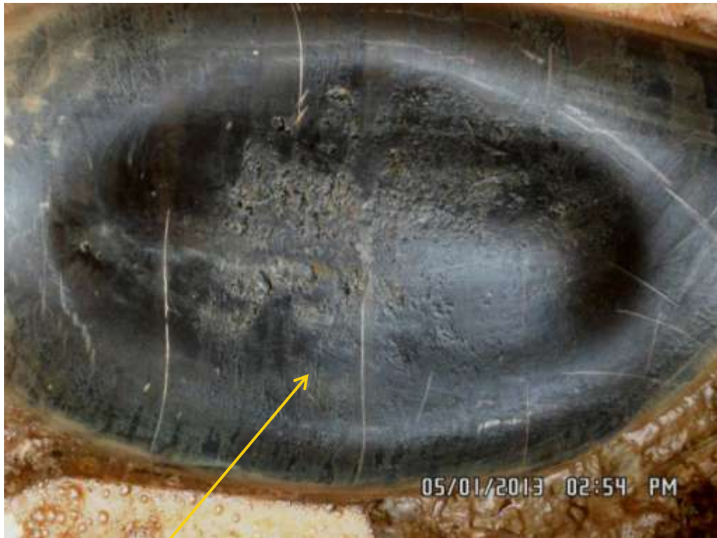
Close up: Depression on 10" Diebu Creek – Nun River pipeline at Onyoma. Picture was taken during Joint Investigation of 5 th January 2013.
