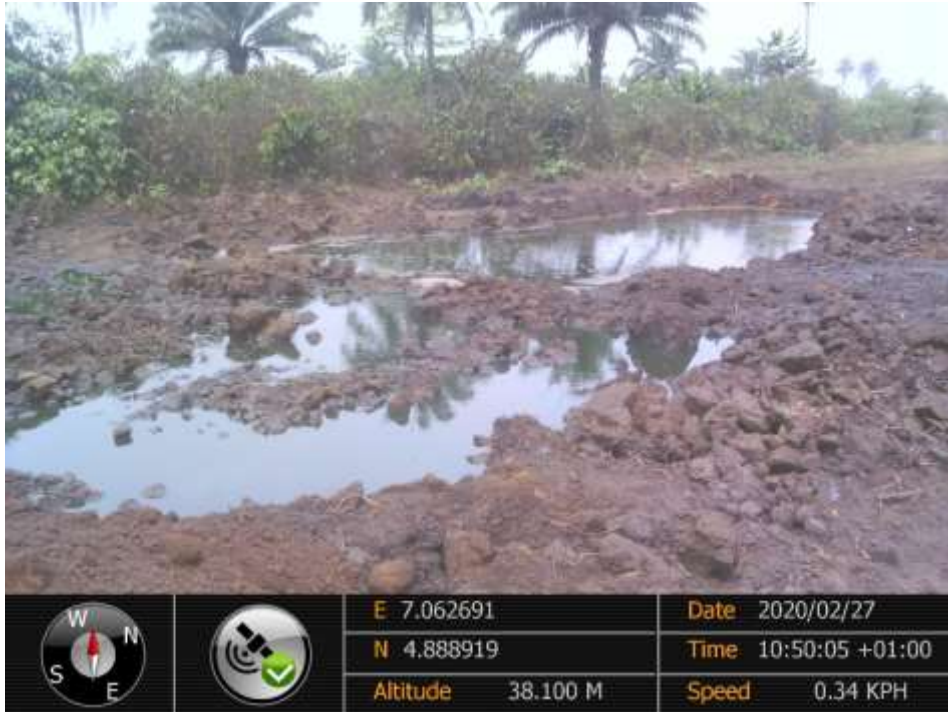
Overview: Part of spill impact on 36inch Nkpoku Bomu Pipeline at Atali . Picture was taken during Joint Investigation of 27 th February 2020.
