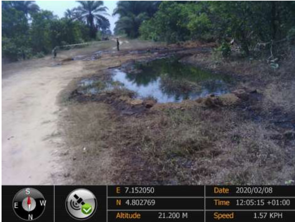
Overview: Part of spill impact on 12" Imo River2 – Ebubu Pipeline at Ogale. Picture was taken during Joint Investigation of 8 th February 2020.
