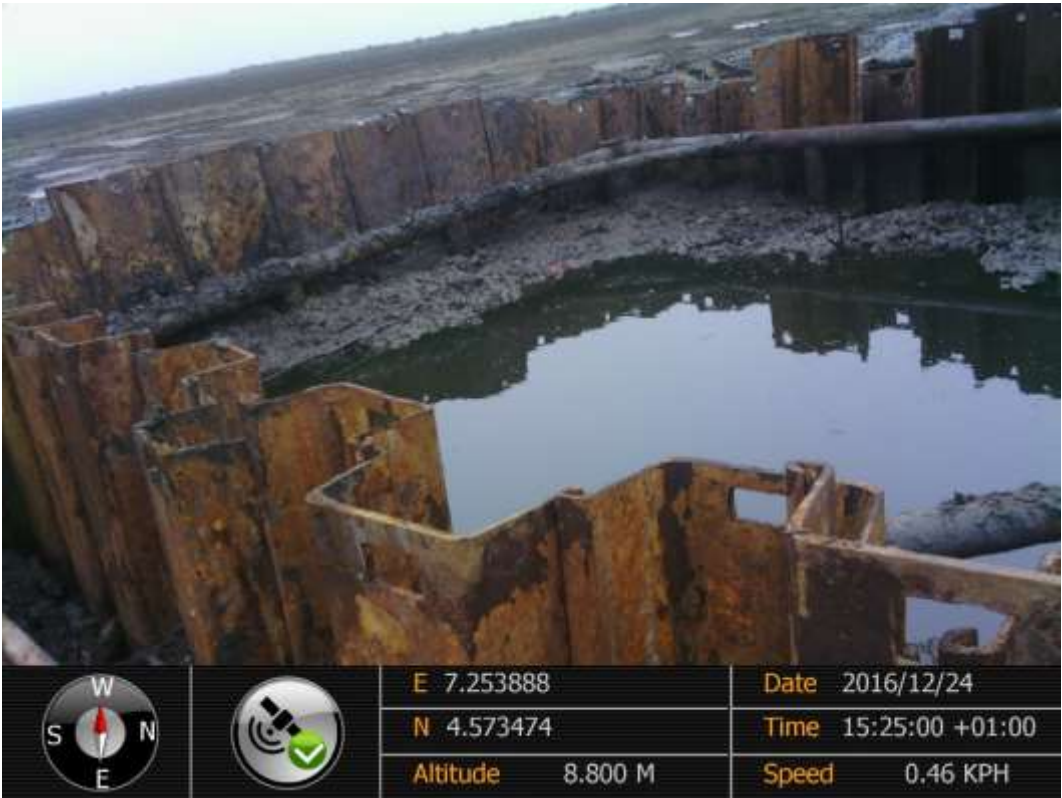
Overview: Spill within cofferdam on 28" Bomu-Bonny Pipeline Right of Way at Bodocity. Picture was taken during Joint Investigation of 24 th December 2016.
