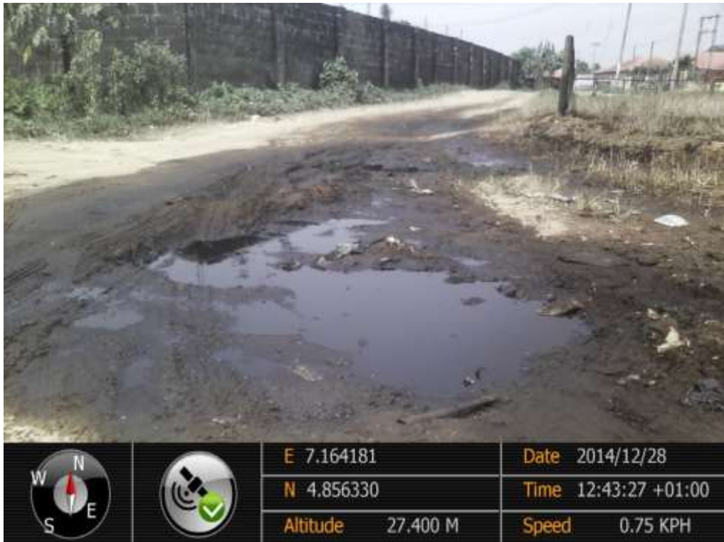
Overview: Part of spill impact on 12" Imo River – Ogale Pipeline Right of Way at KomKom. Picture was taken during Joint Investigation of 28 th December 2014.
