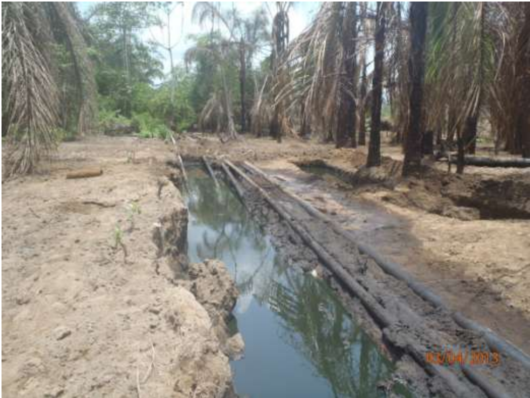
Overview: Part of spill impact on Imo River 4" Well64L flowline right of way at Igiriukwu. Picture was taken during Joint Investigation of 3 rd April 2013.
