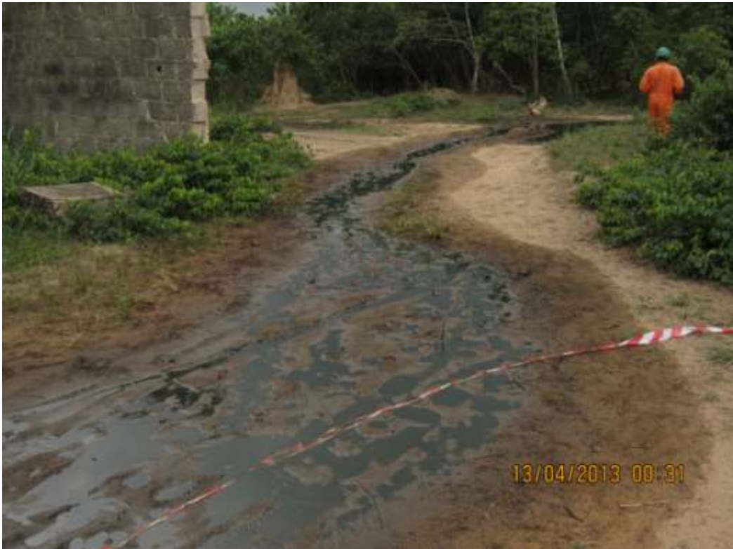
Overview: Part of spill impact on 8" Nkali pipeline right of way at Umuedeokwara. Picture was taken during Joint Investigation of 13 th April 2013.
