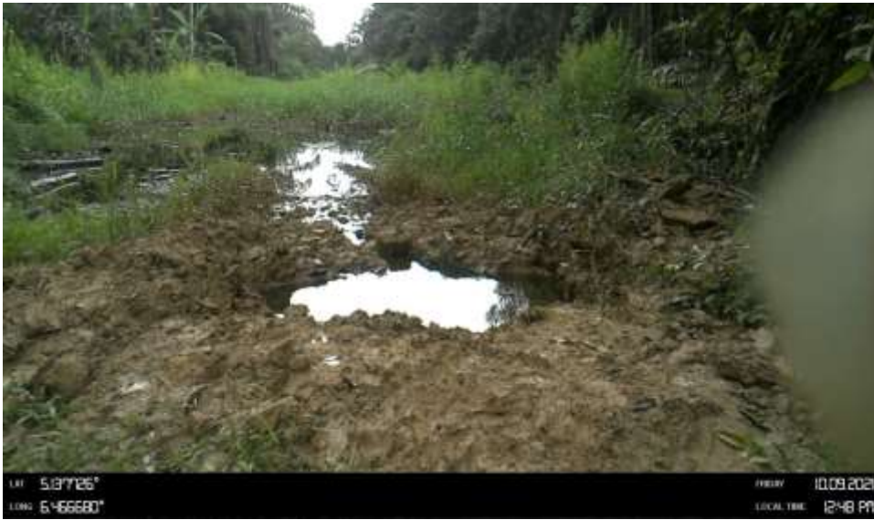
Overview: Part of spill impact on 14" Okordia Rumuekpe Pipeline at Ikarama. Picture was taken during Joint Investigation of 10 th September 2021.
