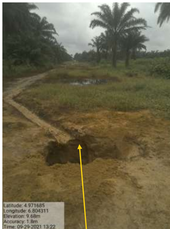
Overview ( Excavated spill point ) : Part of spill impact on 4" Obele Ibaa Delivery line at Ibaa. Picture was taken during Joint Investigation of 29 th September 2021.
