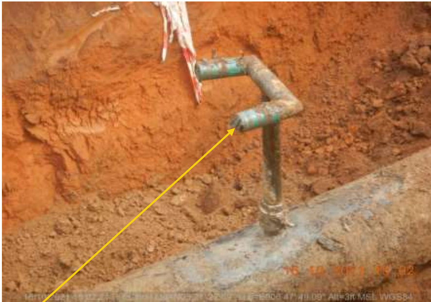
Close-up: Crude oil theft point installed at 12 o'clock position on 18" Assa Rumuekpe Pipeline at Ochia. Picture was taken during Joint Investigation of 13 th October 2021.
