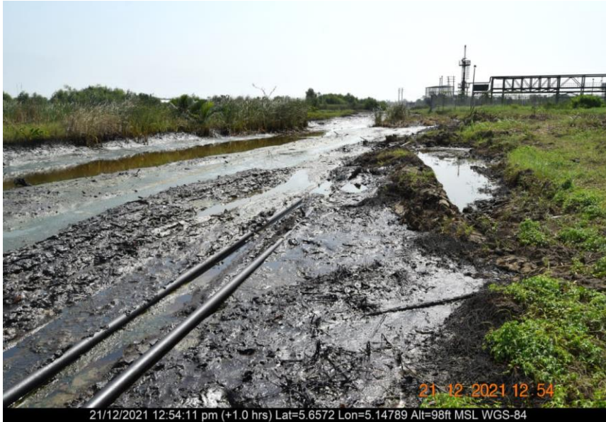
Overview: Part of spill impact on 4" Otumara Well 29S Flowline at Otumara. Picture was taken during Joint Investigation on 21 st December 2021.
