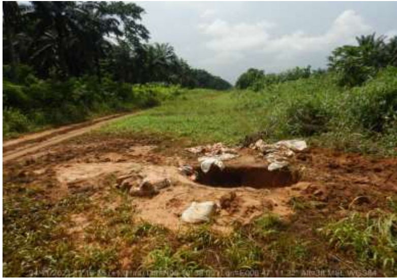
Overview: Part of spill impact on 18" Assa Rumuekpe Pipeline at Umuodibe. Picture was taken during Joint Investigation of 24 th November 2021.
