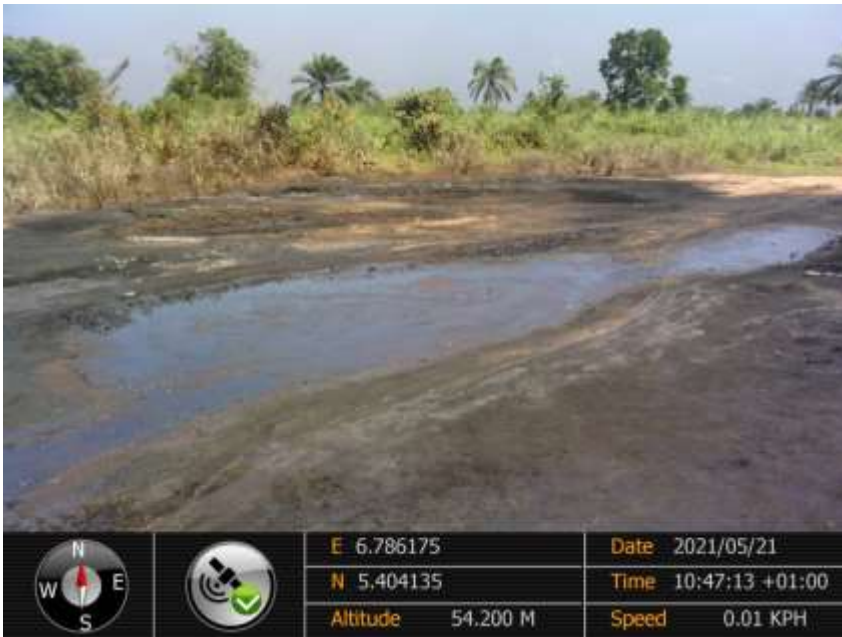
Overview: Part of spill impact on 16inch Egbema Assa Pipeline at Obile. Picture was taken during Joint Investigation of 21 st May 2021.
