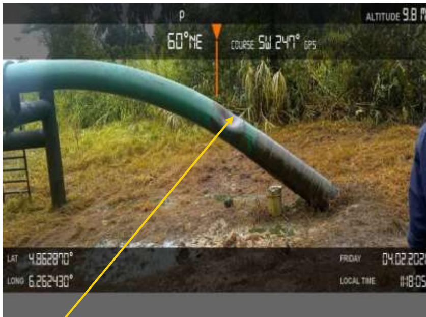
Overview: Part of spill impact on 16inch Nun-River Kolocreek BVS riser at Agbura-Otuokpoti. Picture was taken during Joint Investigation of 2 nd April 2021.
