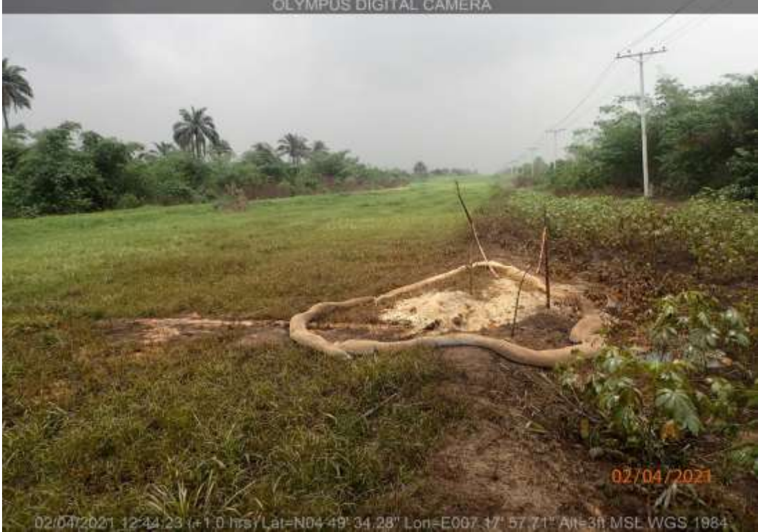
Overview: Part of spill impact on 8inch Afam Well 27T Flowline at Egberu Picture was taken during Joint Investigation of 2nd April 2021 .
