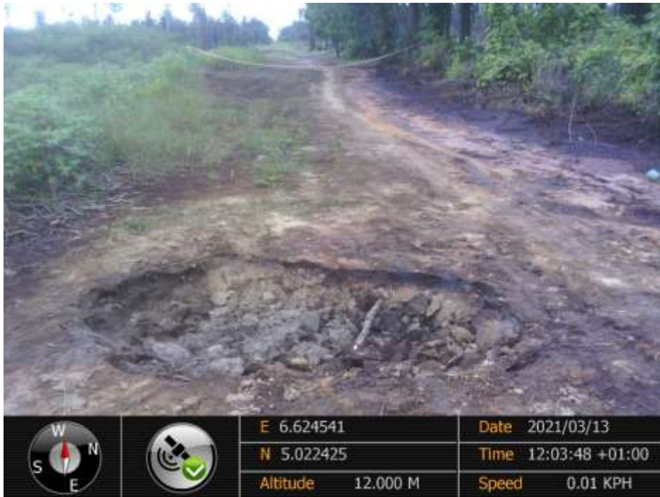
Overview: Part of spill impact on 14inch Okordia Rumuekpe Pipeline at Edeoha. Picture was taken during Joint Investigation of 13 th March 2021.
