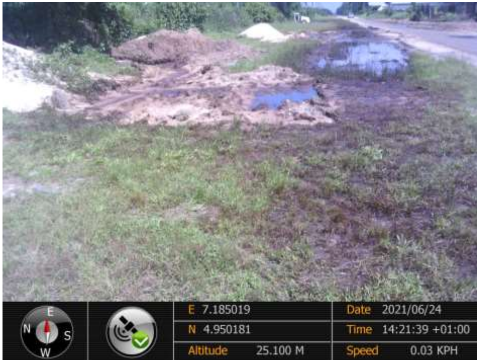
Overview: Part of spill impact on 12inch Imo River 1 – Ogale Pipeline at Owaza. Picture was taken during Joint Investigation of 24 th June 2021.
