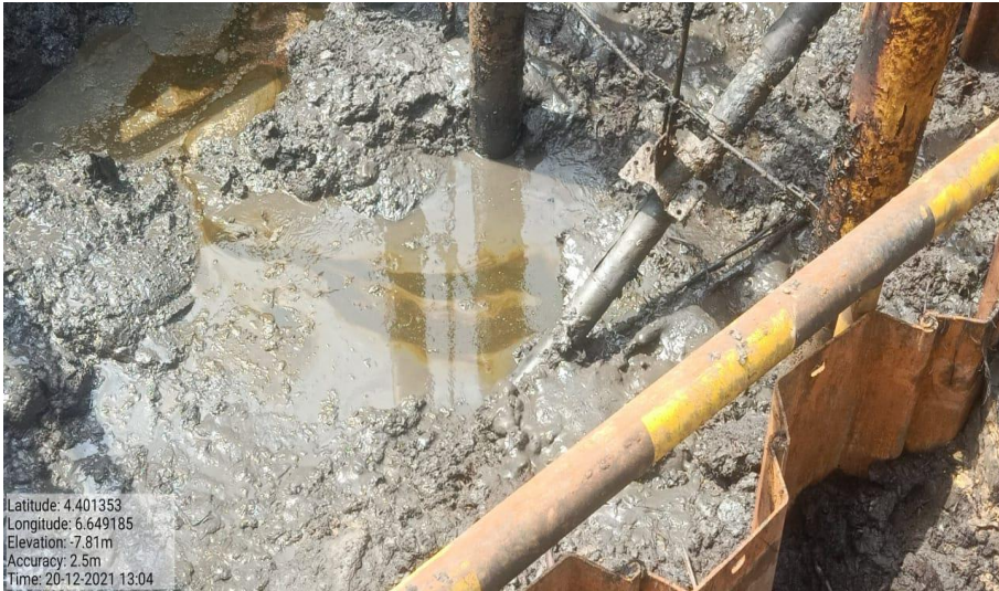
Overview: Part of spill impact on 6'' Belema Delivery line Right of Way at Belema. Picture was taken during Joint Investigation of 20 th December 2021.
