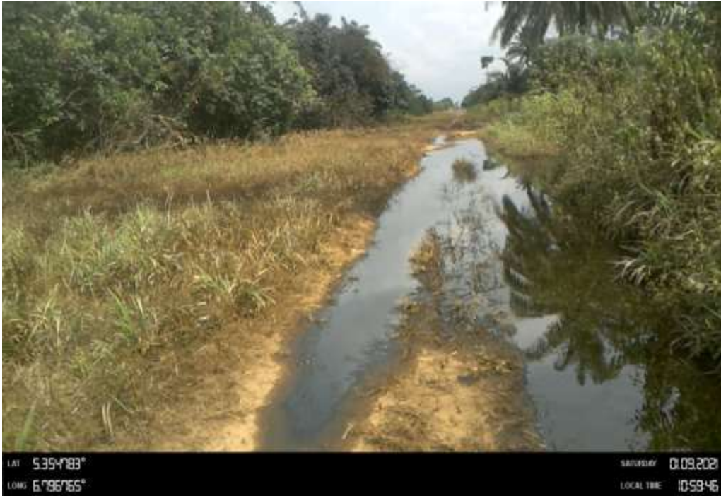
Overview: Part of spill impact on 18inch Assa Rumuekpe Pipeline at Ububo Ochia. Picture was taken during Joint Investigation of 9 th January 2021.
