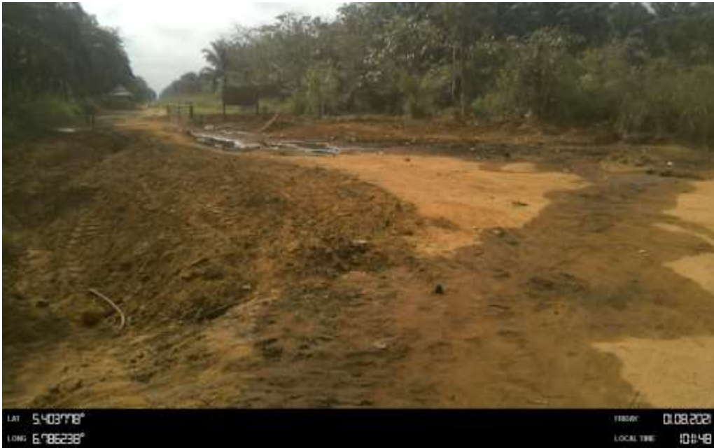
Overview: Part of spill impact on 16inch Egbema Assa Pipeline at Obile. Picture was taken during Joint Investigation of 8 th January 2021.
