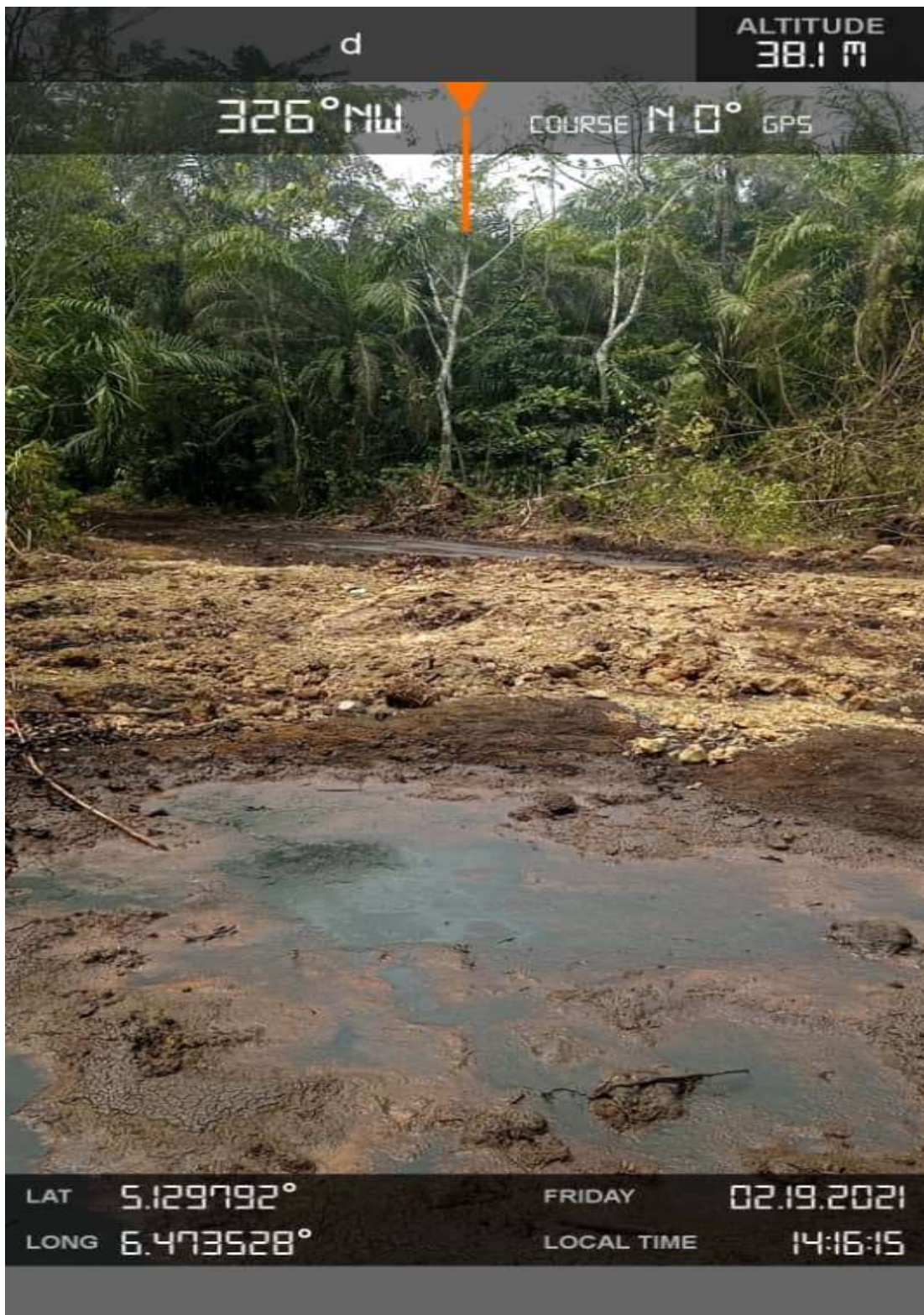
Overview: Part of spill impact on 14inch Okordia Rumuekpe Pipeline at Ikarama . Picture was taken during Joint Investigation of 19 th Feb 2021.
