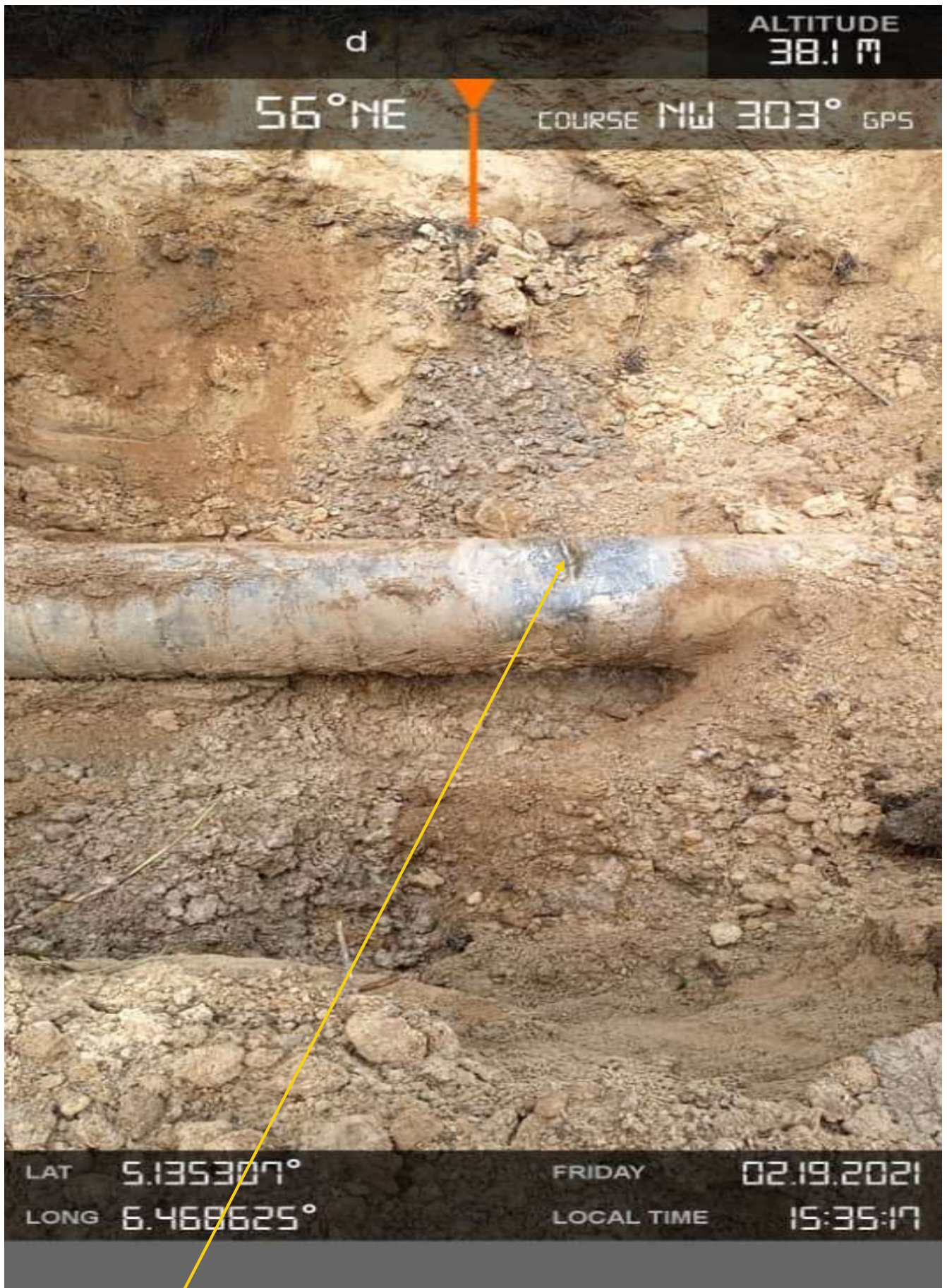
Close-up 3 : Chisel impact with no cut through at point 3 ( 12 o'clock position) on 14inch Okordia Rumuekpe Pipeline at Ikarama . Picture was taken during Joint Investigation of 19 th Feb 2021 .
