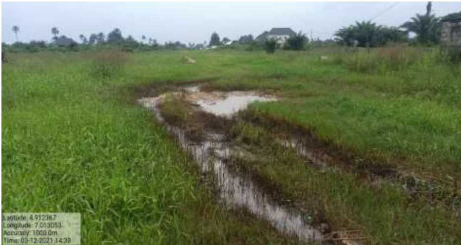
Overview: Part of spill impact on 36" Bomu Bonny Pipeline at Eneka. Picture was taken during Joint Investigation of 3 rd December 2021.
