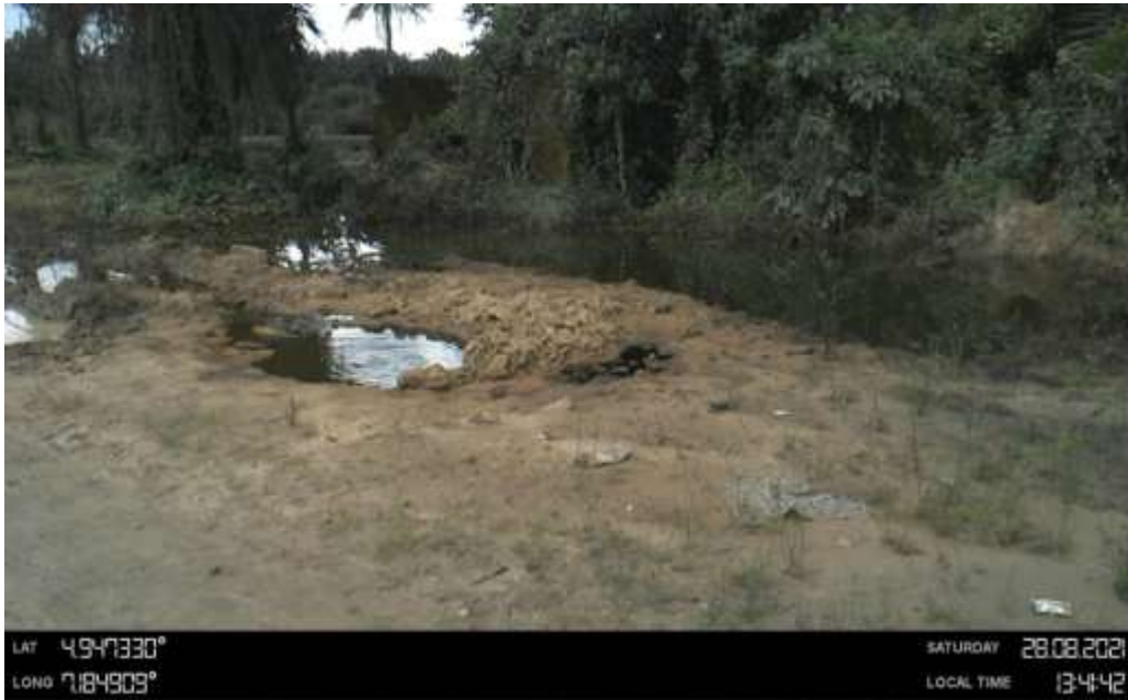
Overview: Part of spill impact on 12" Imo River 2 – Ogale Pipeline at Umulolo. Picture was taken during Joint Investigation of 28 th August 2021.
