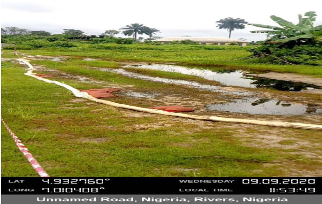
Overview: Part of spill impact on 8" Agbada 2 Nkpoku DeliveryLine at Omuohia - Igwuruta. Picture was taken during Joint Investigation on 9th September 2020.
