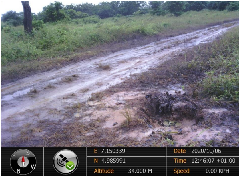
Overview: Part of spill impact on 8'' Nkali ImoRiver 2 Pipeline at Nkali. Picture was taken during Joint Investigation on 6th October 2020.
