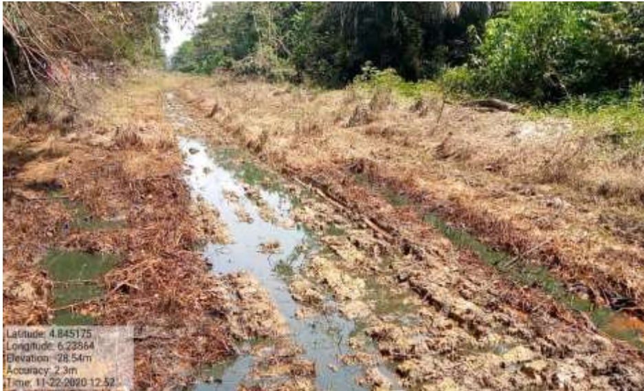
Overview: Part of spill impact on 16inch NunRiver – Kolocreek Pipeline at Otugwe. Picture was taken during Joint Investigation on 22nd November 2020.
