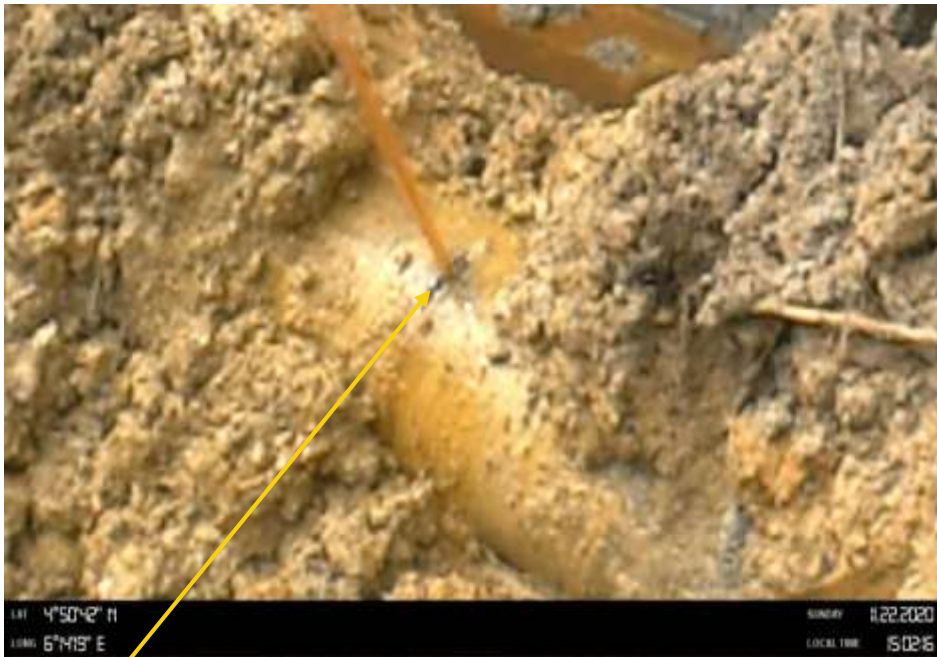
Close-up: Point 1: 2nos hacksaw cut 75m apart at 12 o'clock on 16inch NunRiver – Kolocreek Pipeline at Otugwe. Picture was taken during Joint Investigation on 22nd November 2020.
