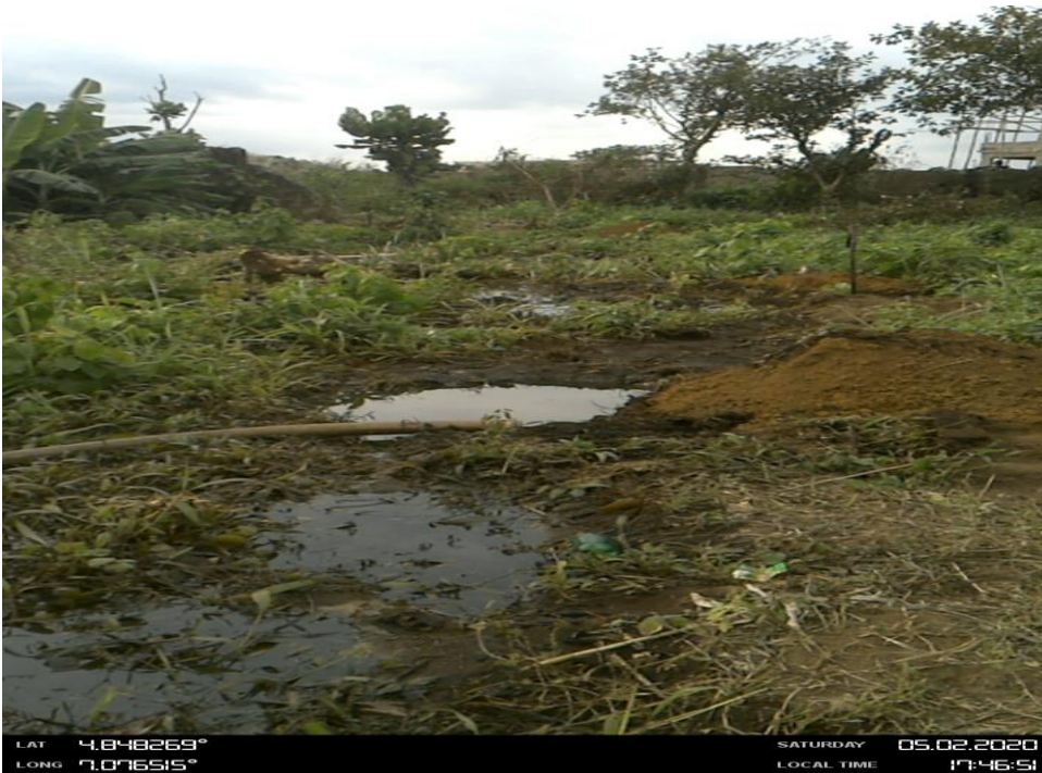
Overview: Part of spill impact on 28" Nkpoku Bomu Pipeline at Elenwo. Picture was taken during Joint Investigation of 2nd May 2020.
