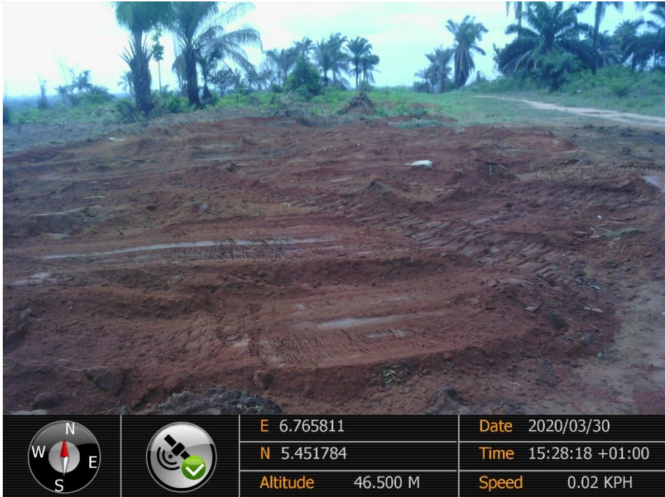
Overview: Part of spill impact on 16" Egbema Assa Pipeline at Umudike. Picture was taken during Joint Investigation of 30 th March 2020.
