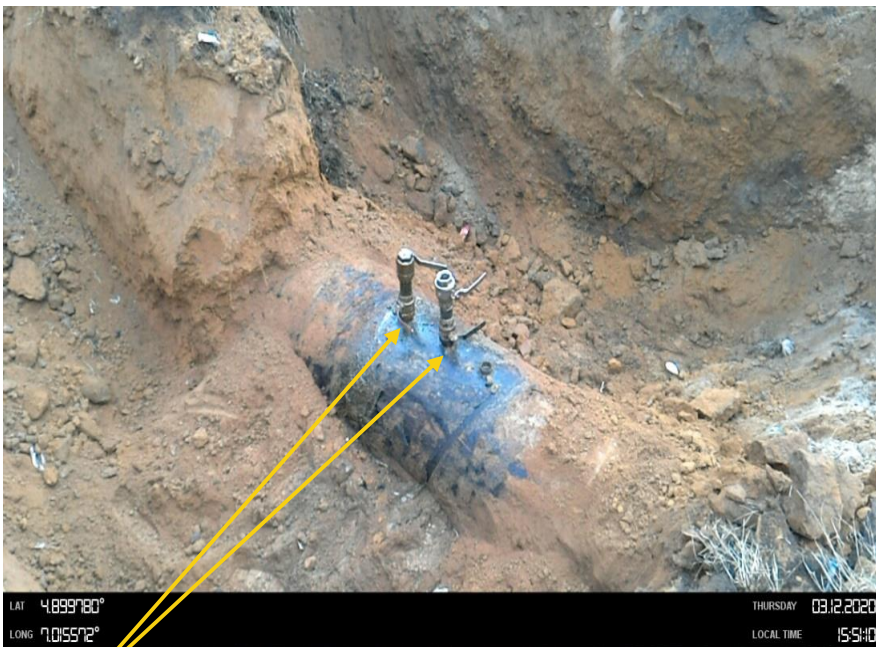
Close-up: 2'' valve crude oil theft points installed at 12 o'clock position on 28'' Nkpoku - Ebulu Pipeline at Rumuowha - Eneka. Picture was taken during Joint Investigation of 12 th March 2020.
