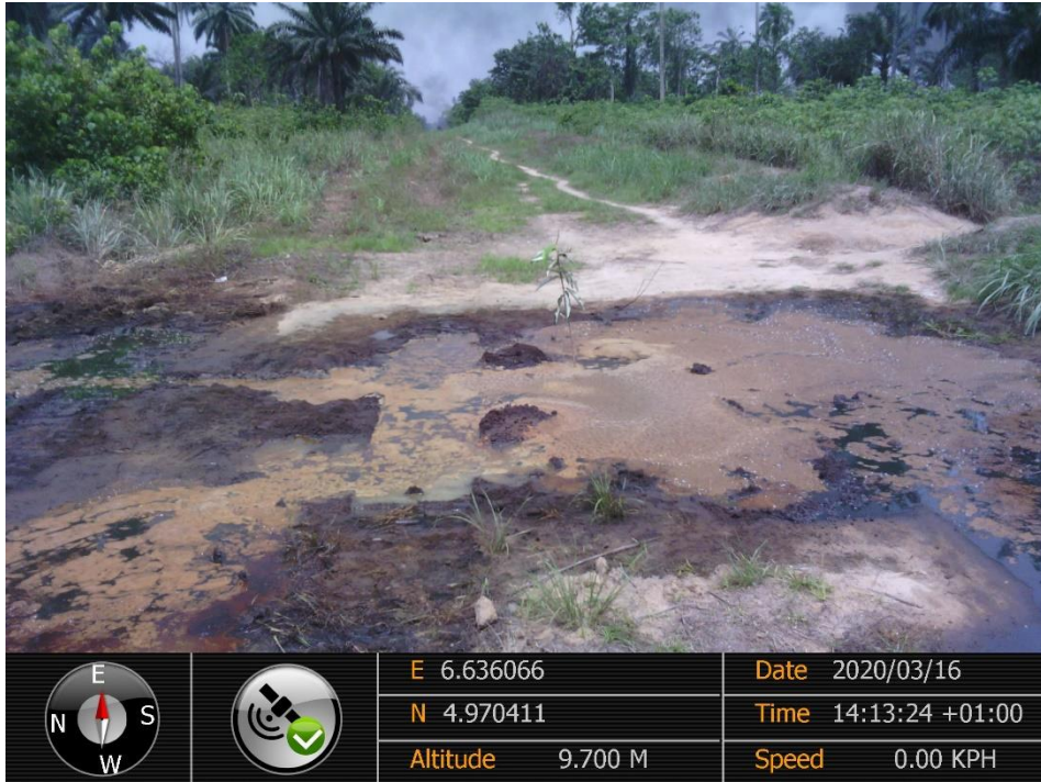
Overview: Part of spill impact on 20" Kolocreek Pipeline Right of Way at Okporowo. Picture was taken during Joint Investigation of 16 th March 2020.
