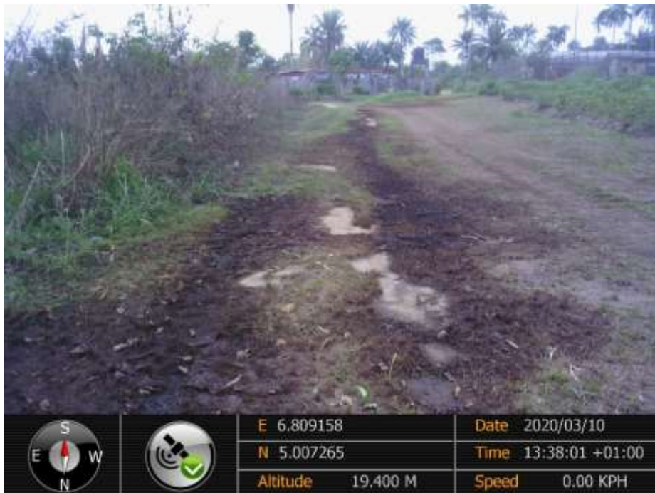
Overview: Overflow from sump-pit on Obele Flow station at Obele. Picture was taken during Joint Investigation of 10 th March 2020.
