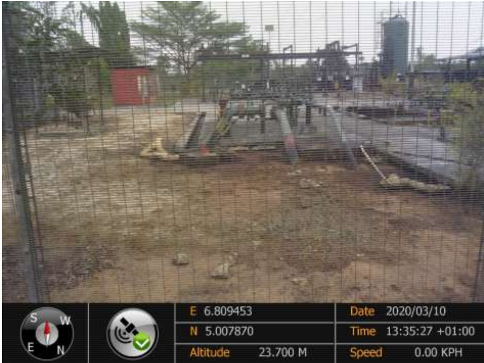
Overview: Part of spill impact around Obele Flow station at Obele. Picture was taken during Joint Investigation of 10 th March 2020.
