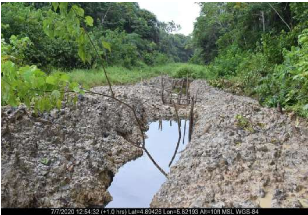
Overview: Part of spill impact on 8" Seibou-Ajatiton Bulklineat Agbidiamma. Picture was taken during Joint Investigation 7th July 2020.
