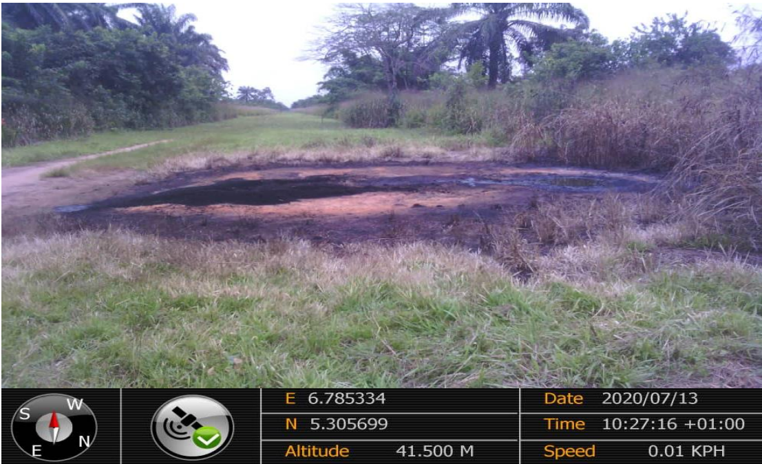
Overview: Part of spill impact on 18" Assa - Rumuekpe Pipeline at Awara. Picture was taken during Joint Investigation 13th July 2020.
