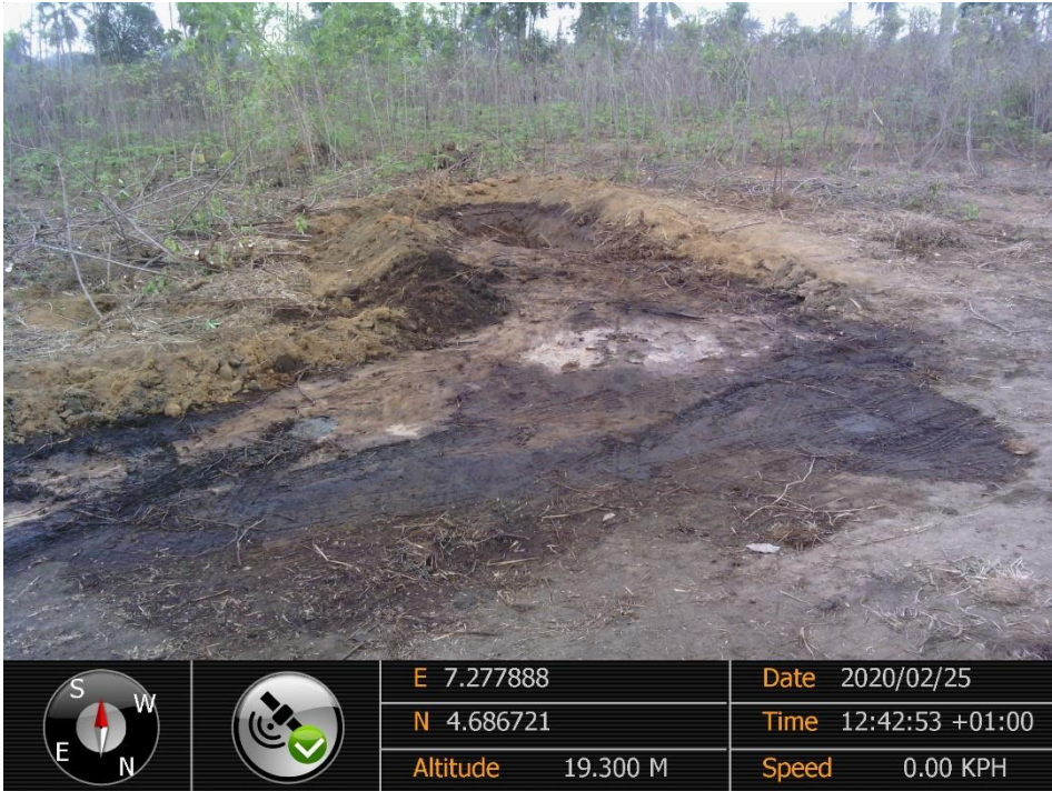
Overview: Part of spill impact on 24" Ogale – Bomu Pipeline Right of Way at Biara . Picture was taken during Joint Investigation of 25 th February 2020.
