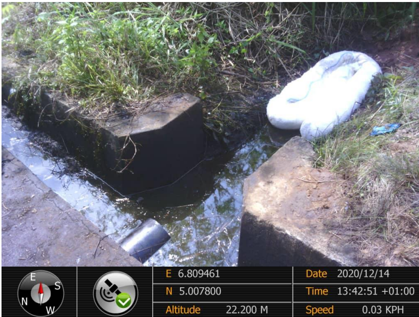
Close-up: Saver pit overflow from drainage on Obele flowstation at Obele. Picture was taken during Joint Investigation on 14 th December 2020.
