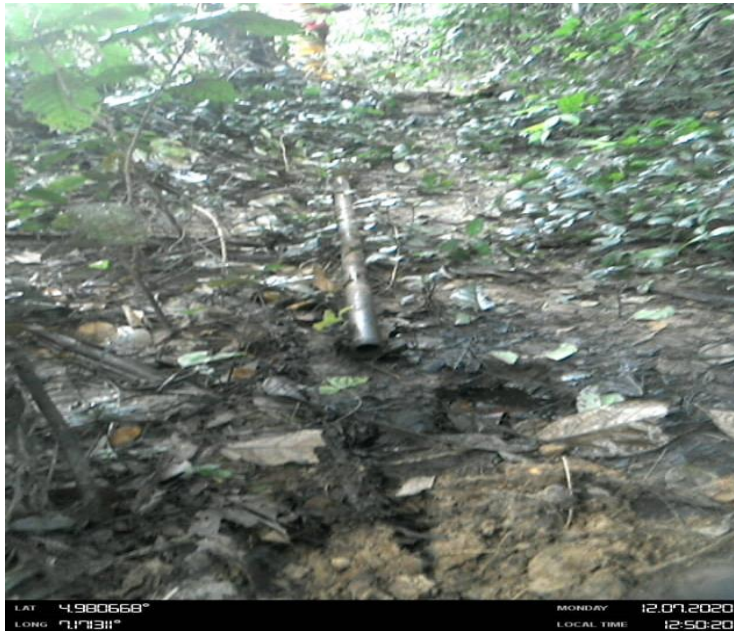
Overview: Part of spill impact on 4" ImoRiverWell 60T Flowline at Odagwa. Picture was taken during Joint Investigation on 7th December 2020.
