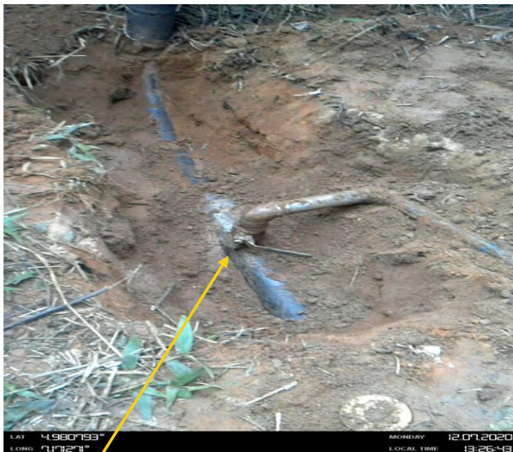
Close-up: Crude oil theft point installed at 12 o'clock position on 4" ImoRiverWell 60T Flowline at Odagwa. Picture was taken during Joint Investigation on 7th December 2020.
