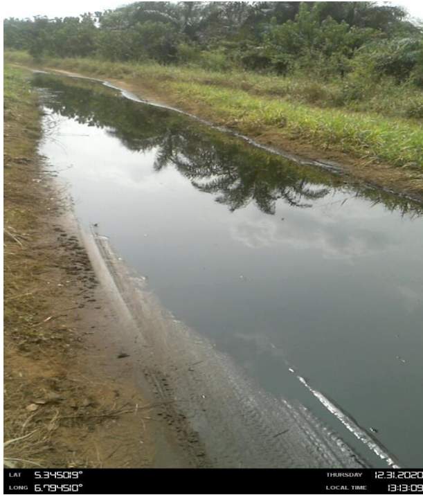
Overview: Part of spill impact on 18" Assa - Rumuekpe Pipeline Right of Way at Ochia. Picture was taken during Joint Investigation of 31 st December 2020.
