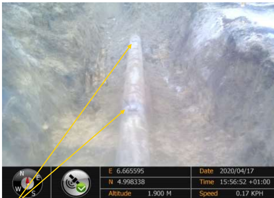
Close-up: 2nos 3" weld neck flang crude theft points at 12 o'clock position on 14" Okordia – Rumuekpe Pipeline at Ihunwo. Picture was taken during Joint Investigation of 17 th April 2020.
