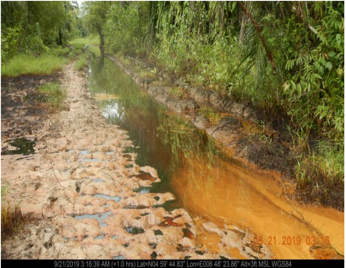
Overview: Part of spill impact on 4" Obelle - Ibaa Pipeline Right of Way at Ibaa. Picture was taken during Joint Investigation of 21 st September 2019.
